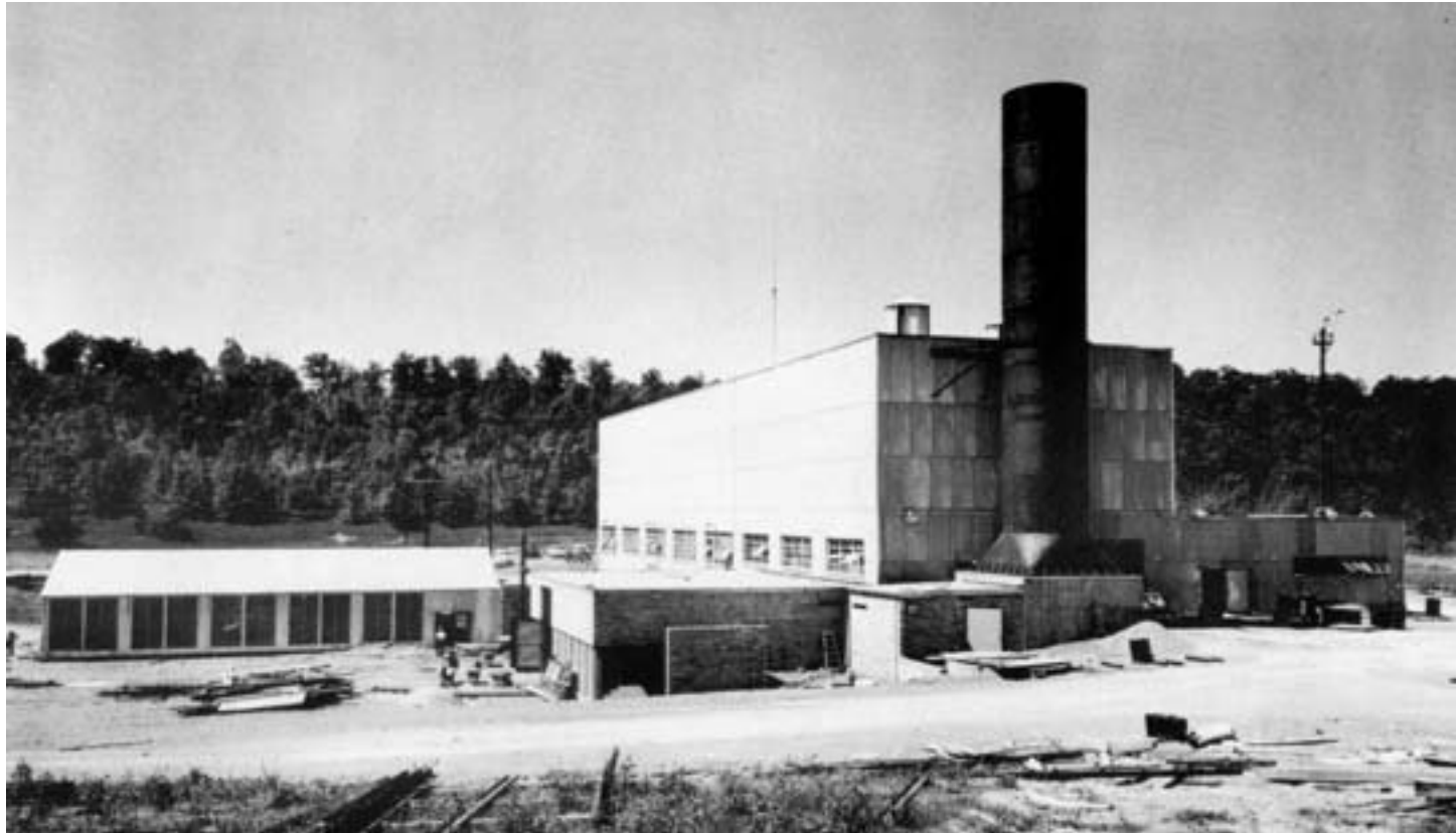
Bldg. 7303, Oak Ridge National Laboratory
